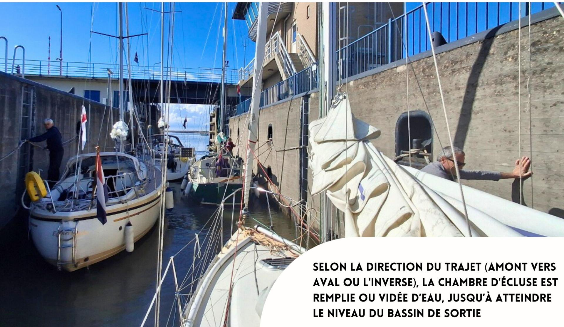
SELON LA DIRECTION DU TRAJET (AMONT VERS AVAL OU L'INVERSE), LA CHAMBRE D'ÉCLUSE EST REMPLIE OU VIDÉE D'EAU, JUSQU'À ATTEINDRE LE NIVEAU DU BASSIN DE SORTIE
